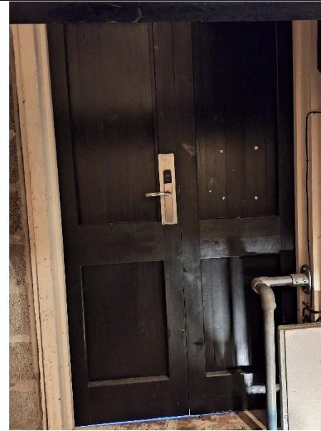
Salto access door out onto roof
