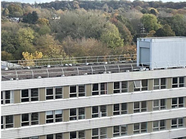
5 th floor block roof
