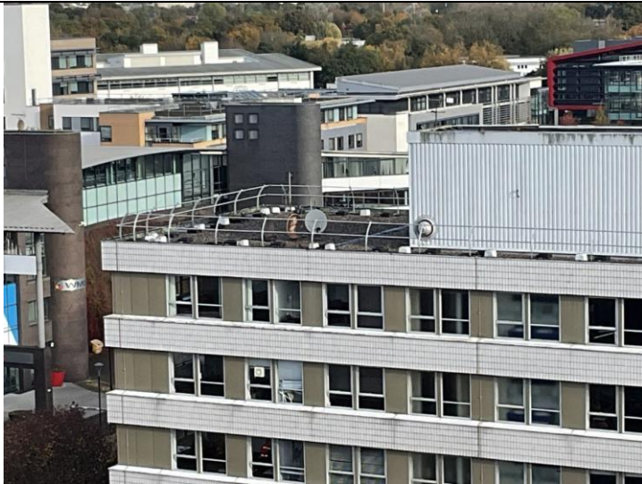
5 th floor block roof
