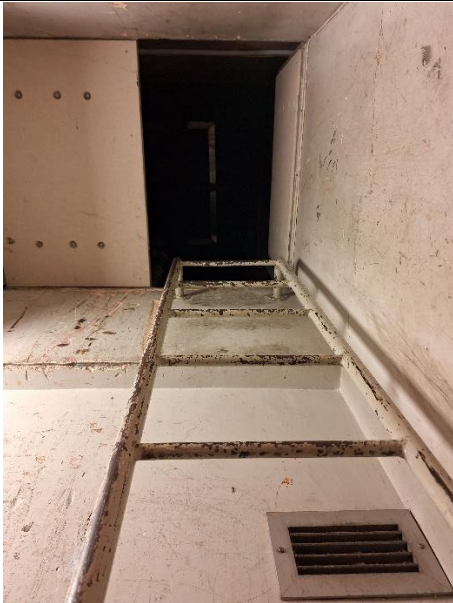
Ladder access to rooftop plant room
