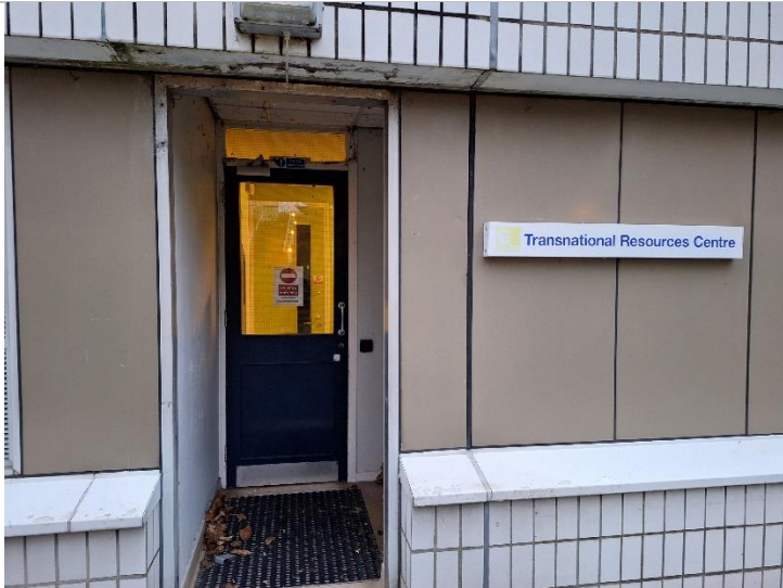
Side entrance for lower roof access
