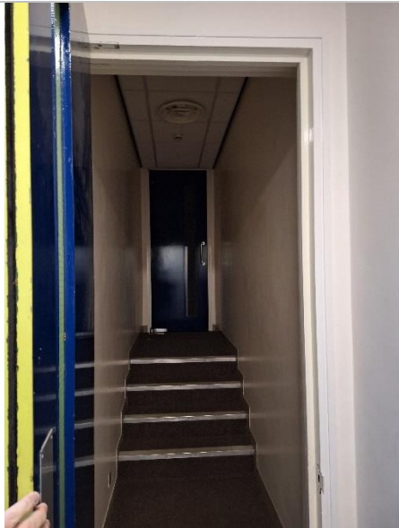
Corridor leading to plantroom
