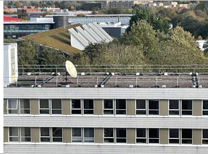
5 th floor block roof
