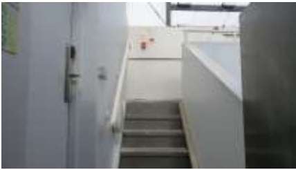
South access to the internal gantry
