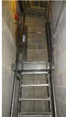
South Entrance staircase to roof
