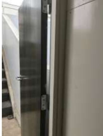
2 nd Door leading to North roof access. No Salto access required.
