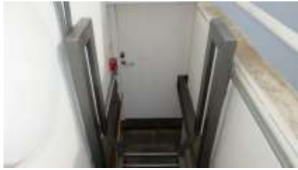
Access to North roof from internal gantry
