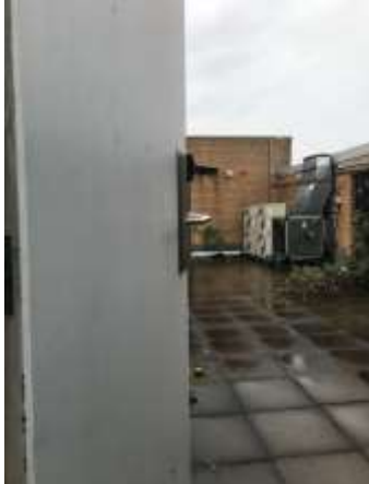
Door with Salto access leading to North roof staging area
