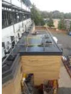
Lower level roof
