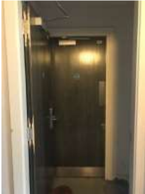
South Entrance (Salto Required) on first door
