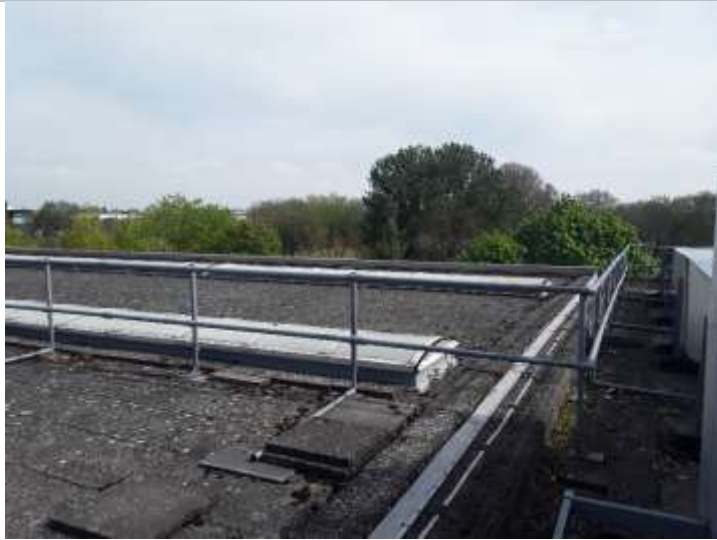
General edge protection around parts of roof
