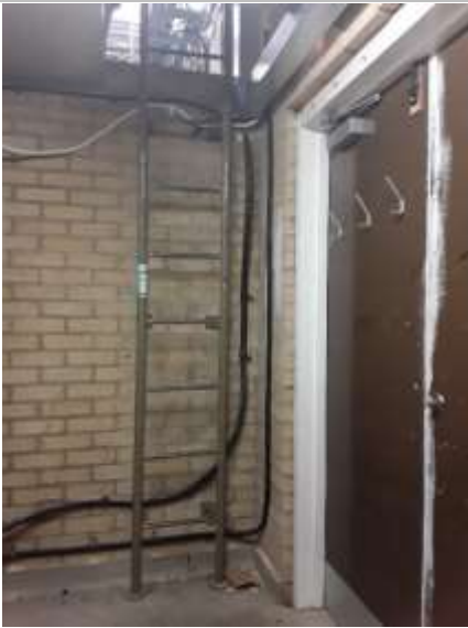
Roof access ladder
