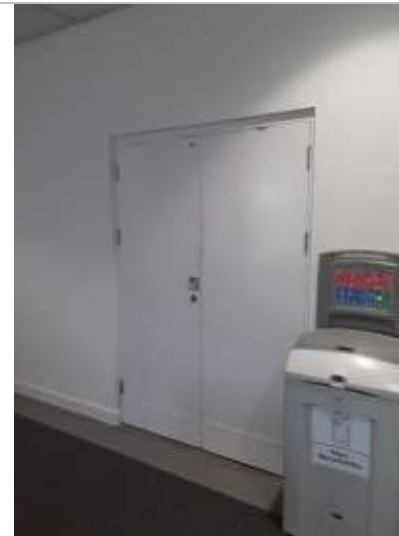
Roof ladder access door (S1 key required)
