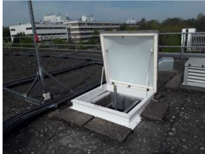
Hatch out onto roof
