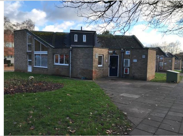
Whitefields roof view front elevation
