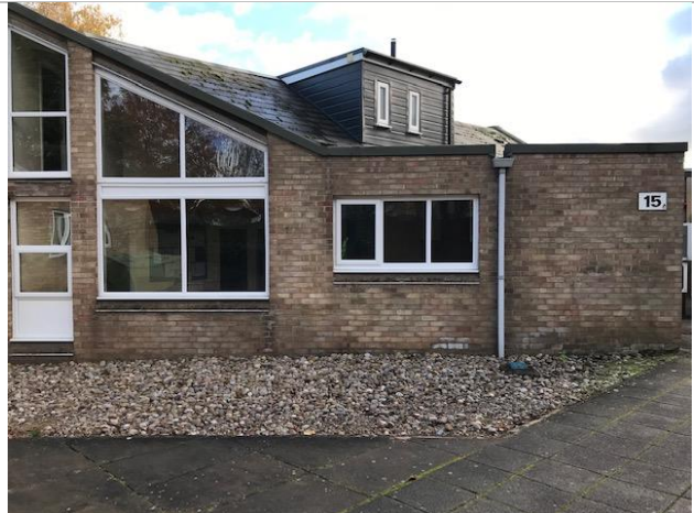
Whitefields roof view front elevation
