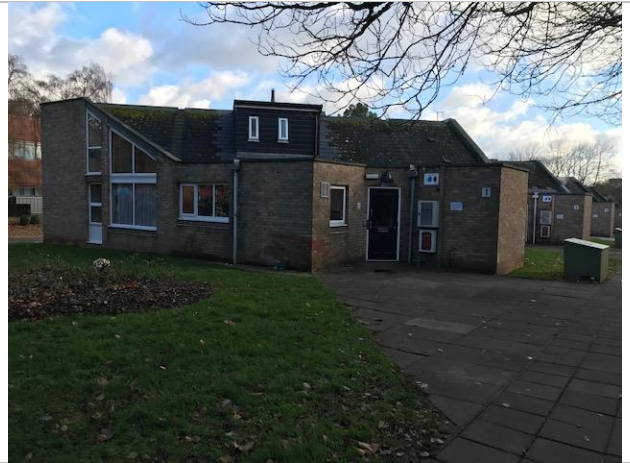
Whitefields roof view front elevation
