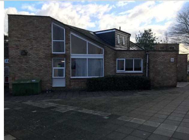
Whitefields roof view side elevation
