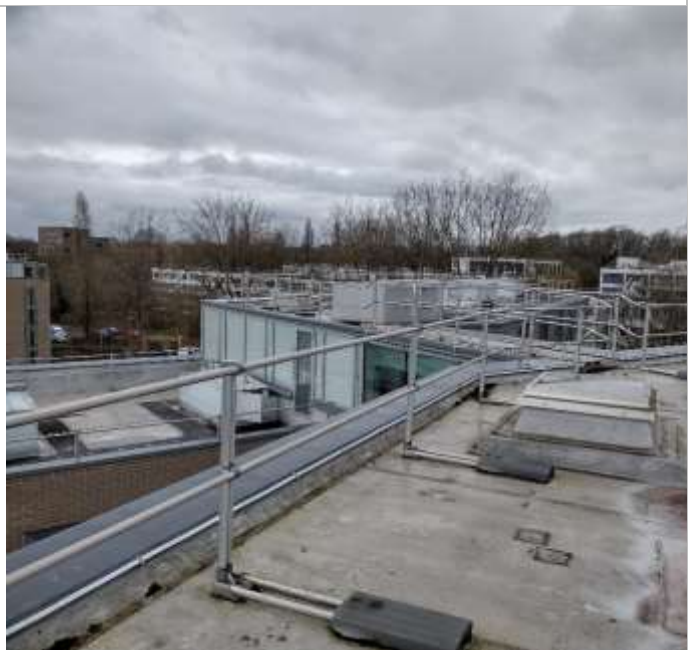
Skylights and hatches situated on the roof space.
