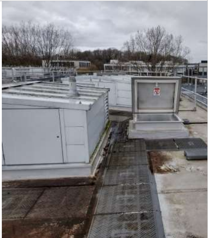
The roof space has designated walkways.
