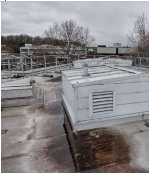
The roof space benefits from edge protection.
