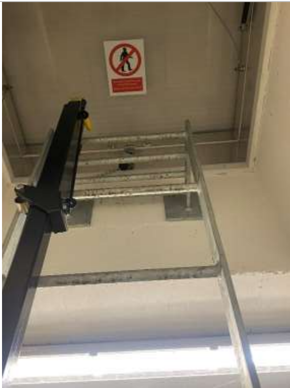
Go up through the roof hatch on to the roof space.
