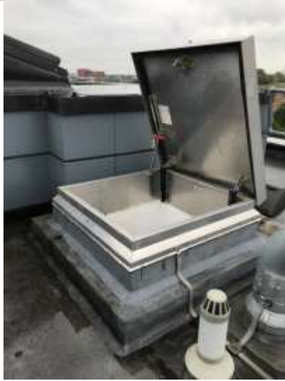
Roof Hatch with Salto Fob
