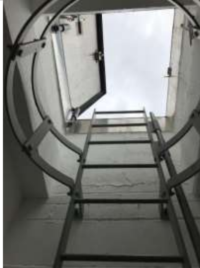
Galvanised loop ladder leading to roof hatch
