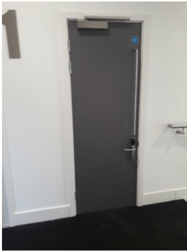
First floor internal access door
