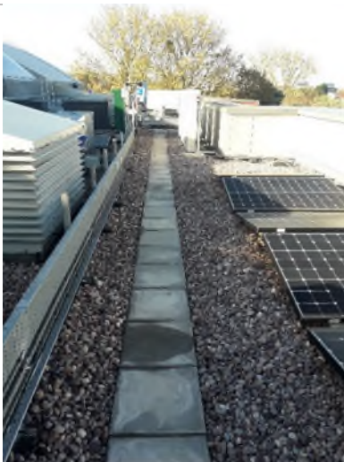
Flat roof walkway and plant
