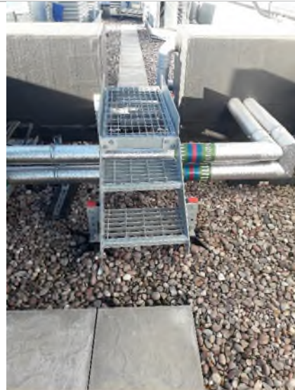
Gantry accessways over plant
