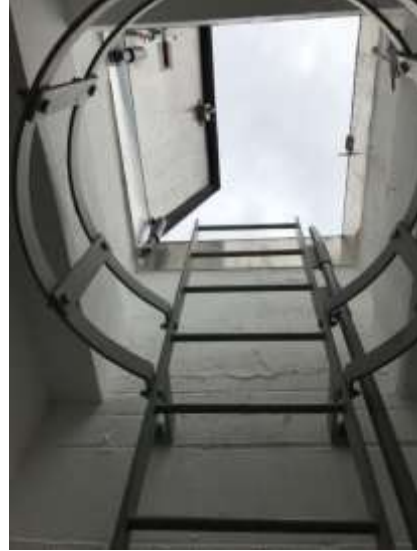
Galvanised loop ladder leading to roof hatch
