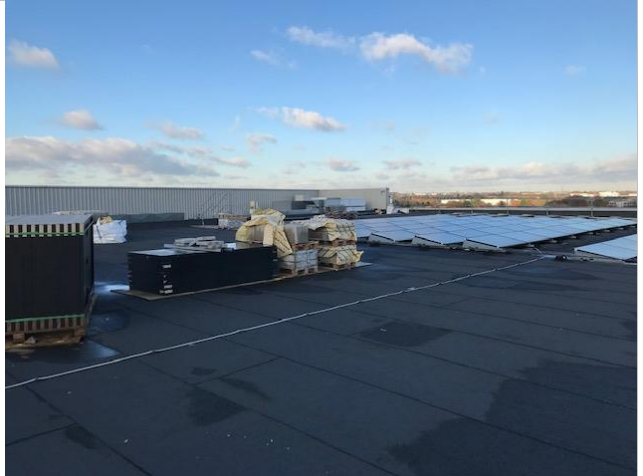
External roof staging area
