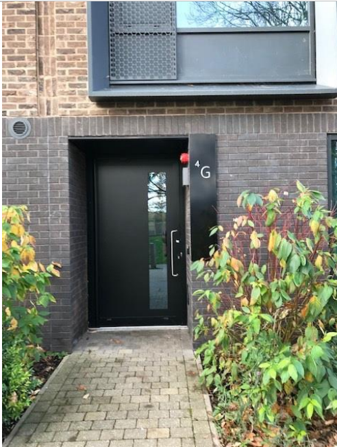
Apartment Cryfield 4G to access the roof
