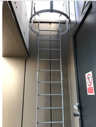
Cryfield 7 access door to roof. Left leads to lower level roof, Galvanised steel ladder leads to higher level roof.
