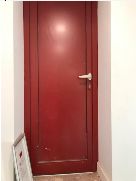
Cryfield 6 door to lower level roof
