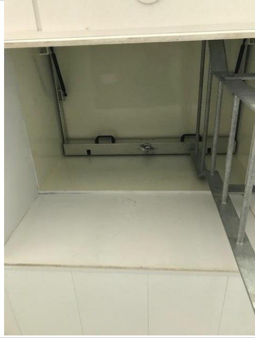
Cryfield 6 roof hatch to higher level roof
