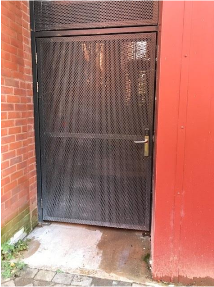
Cryfield 8 External access staircase to roof. Salto access to ground floor and second floor gate.
