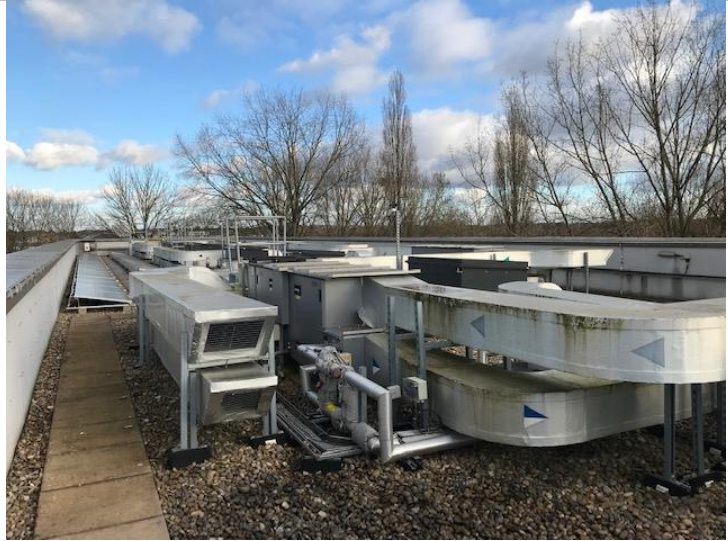
Cryfield 5 External roof
