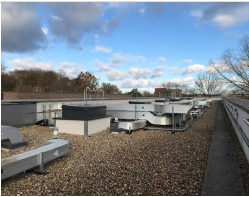
Cryfield 5 External roof
