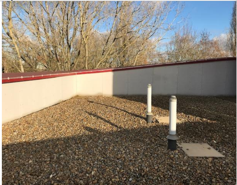
Cryfield 6 lower level external roof
