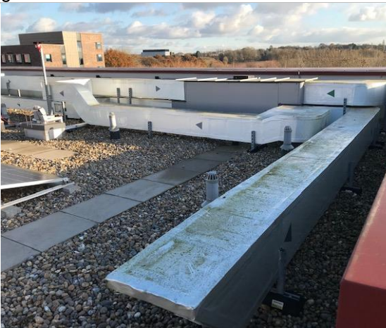
Cryfield 8 External roof
