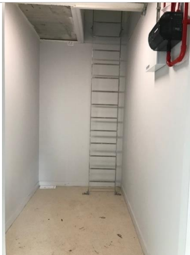
Cryfield 9, galvanised fixed vertical ladder leading to the roof hatch
