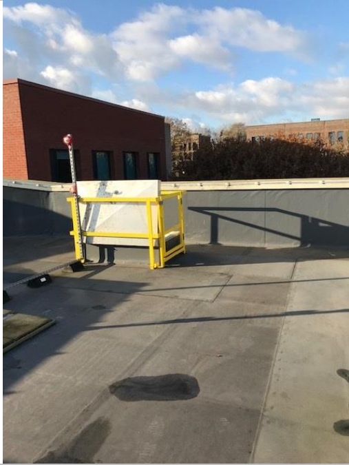
Cryfield 9 External roof
