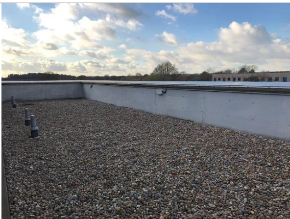
Cryfield 7 Lower external roof
