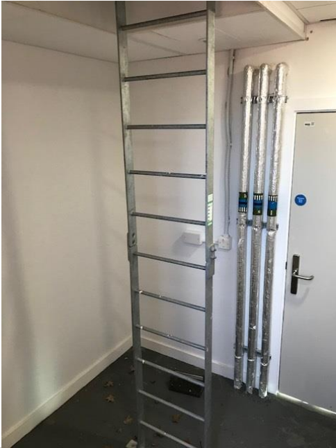
Cryfield 6 fixed galvanised steel ladder leading to the higher level roof
