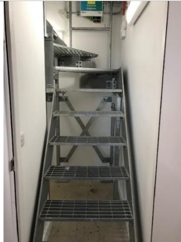
Cryfield 4 Galvanised stairs leading to the roof
