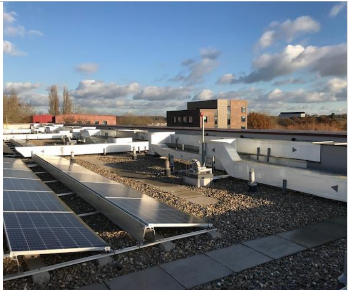
Cryfield 8 External roof.
