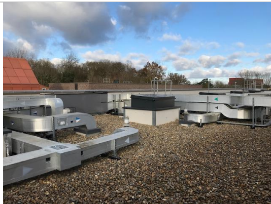
Cryfield 5 External roof
