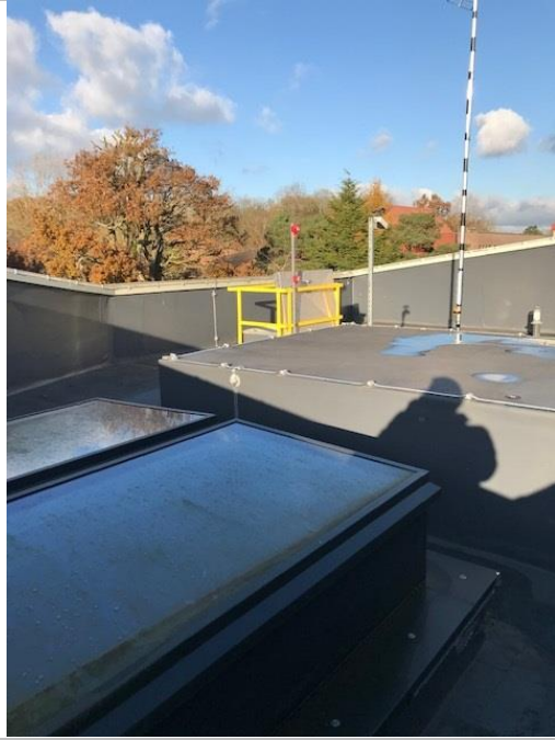
Cryfield 9 External roof
