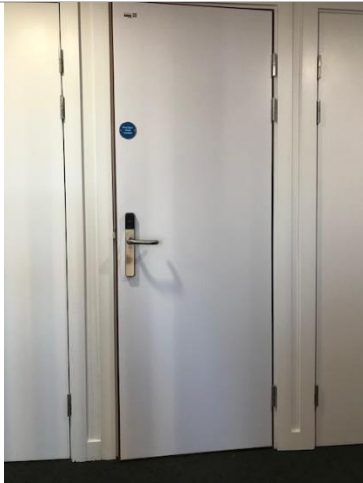
Cryfield 4 Access door to roof with Salto fob
