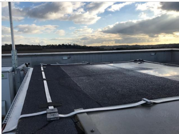
Cryfield 7 Higher external roof
