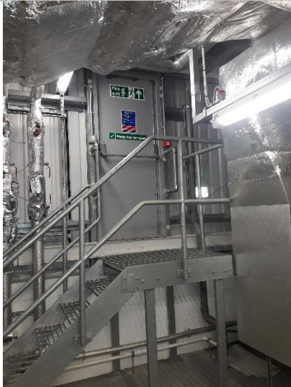
Roof access door leading out onto higher level roof (Salto)
