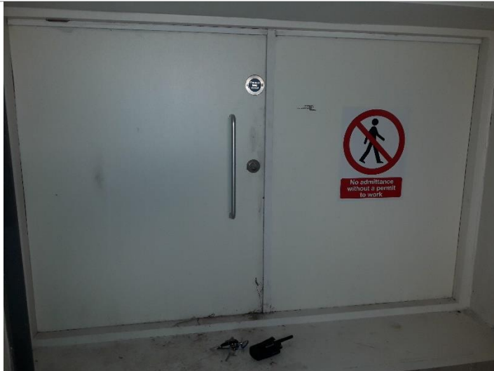
Example of hatch type door leading out onto roof (Salto)
