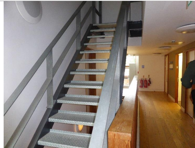
Main stairwell leading to plant room door
