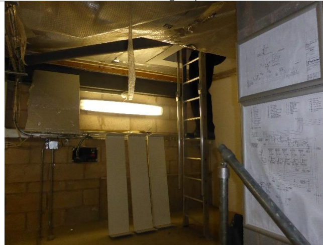
Example of vertical access ladders to roof
