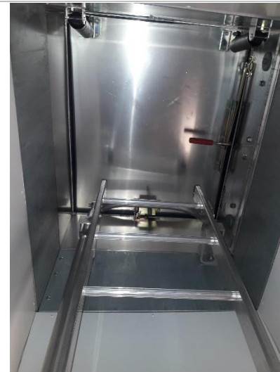
Example of ceiling hatch leading out onto roof (Salto)
