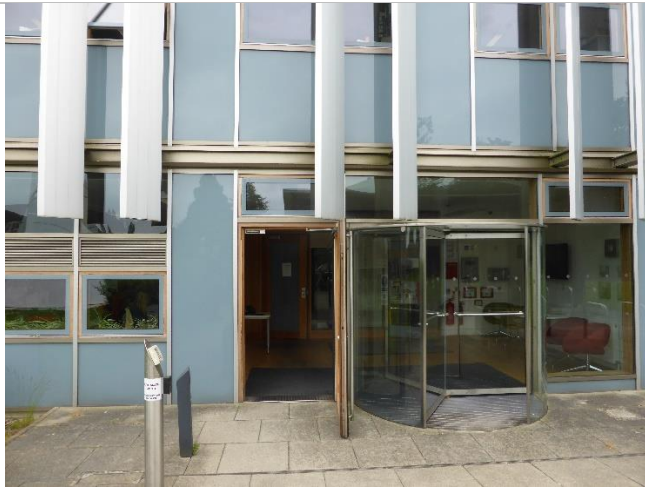
MCCB Main entrance
