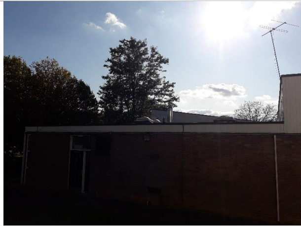
Roof protrusions (Sky light and exhausts/vents)
