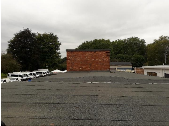
Roof view & no edge protection
