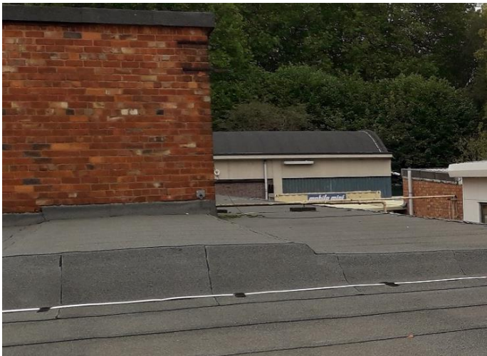
Roof view & no edge protection
