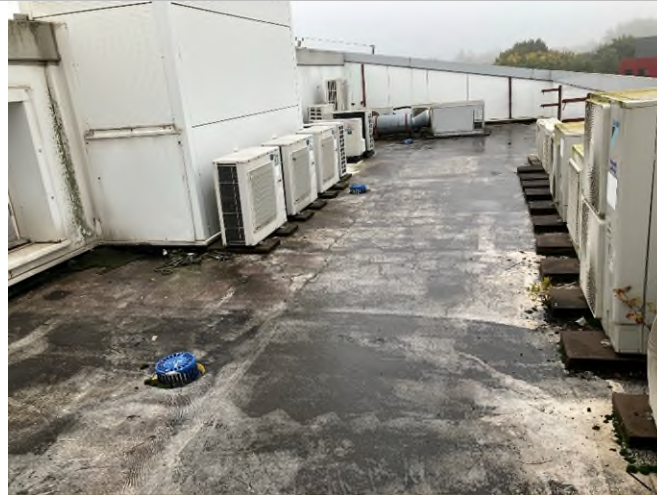
Second section of roof space.
