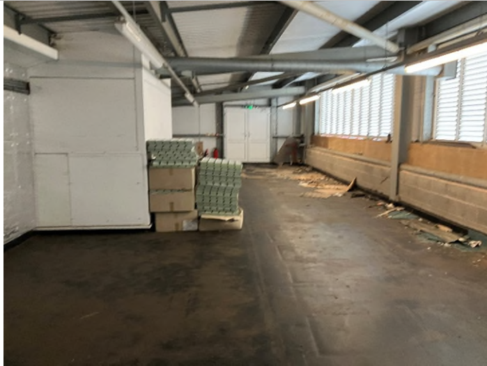
Undercover walkway leading through to other section of flat roof space.
