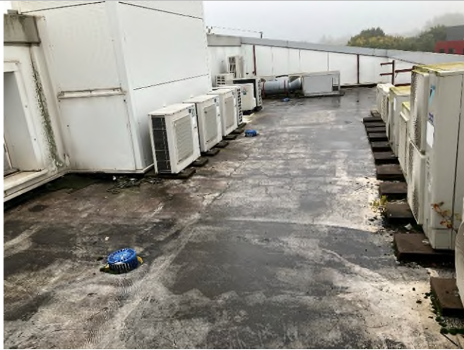
Second section of roof space.
