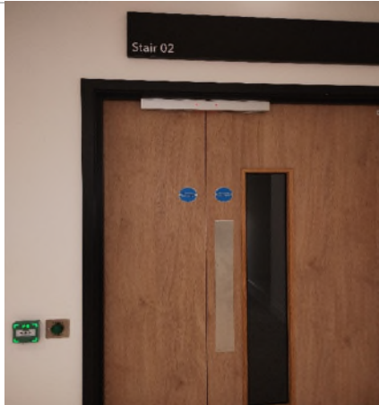
Internal door on ground floor leading to stairwell to rood space
