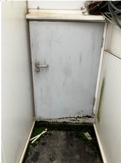
Door hatch that led out onto the roof.
