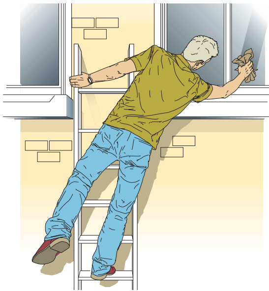
Figure 1a Incorrect - overreaching and not maintaining three points of contact
