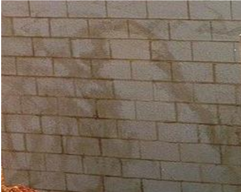
Concrete masonry unit wall
