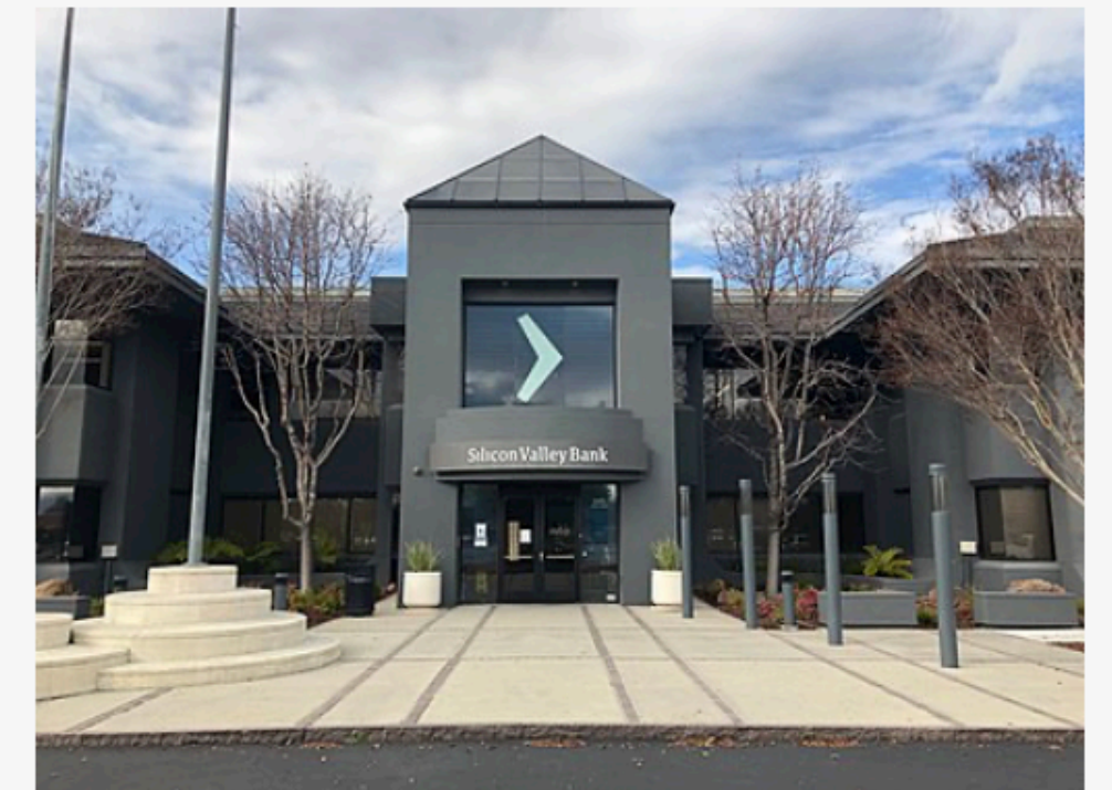
Headquarters in Santa Clara
