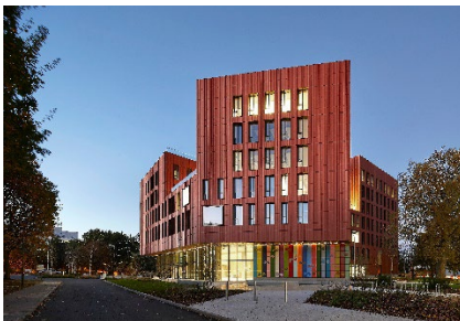
Faculty of Arts Building (FAB)
